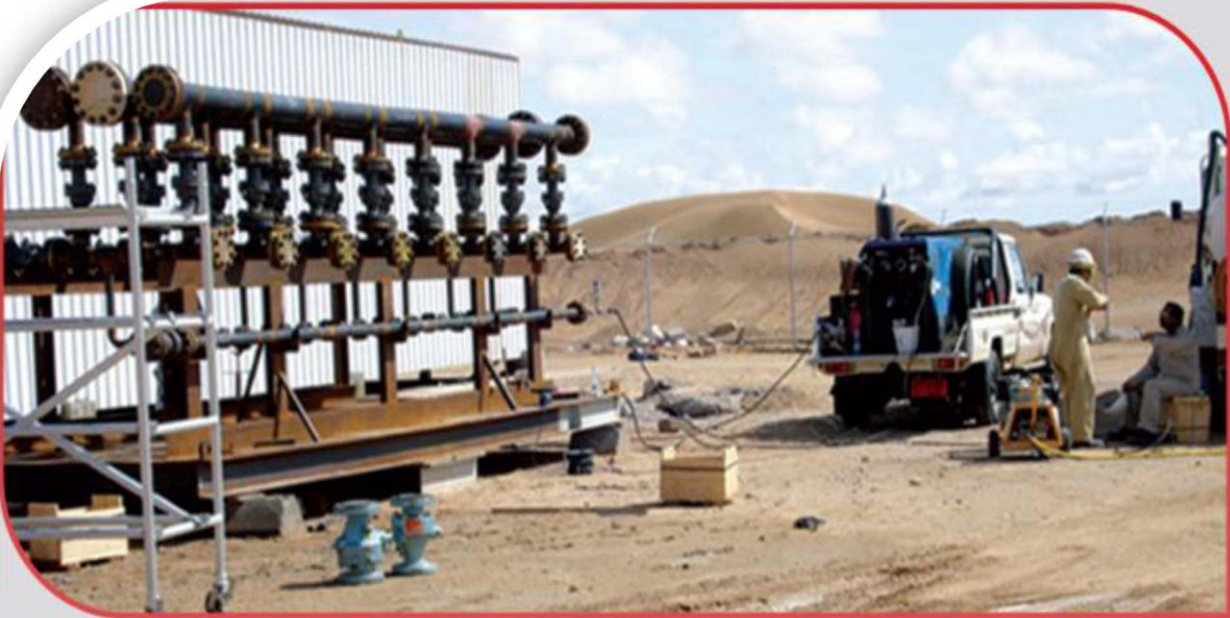
Home Made Manifold That Was Fabricated, Welded, And Installed By Our Welding Crew At Oxy Block S1
